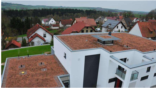
FIGURE6: SHOWS THE MAPEPLAN T INSTALLED ON GREEN ROOF WITH SOIL BALLAST
