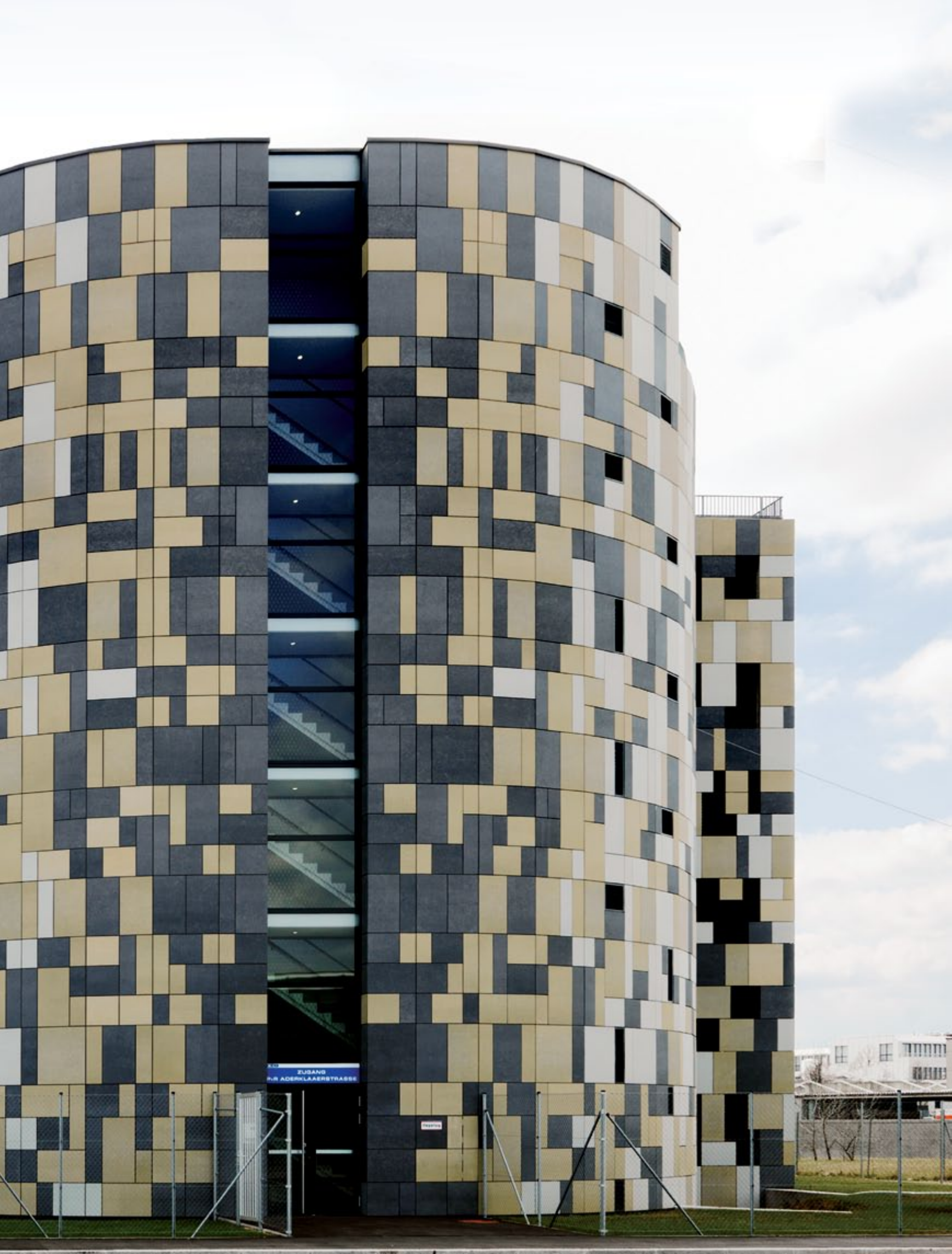
Park & Ride Aderklaa Vienna, AT | AW Architects Vienna, AT | 1,800 m 2 fibreC facade | ivory, sandstone & anthracite | FE, FL & MA | riveted Park & Ride Aderklaa Wien, AT | AW Architekten Wien, AT | 1.800m 2 fibreC Fassade | elfenbein, sandstein & anthrazit | FE, FL & MA | genietet
