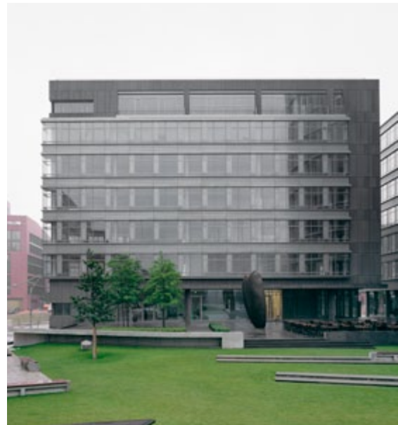
Bavaria Office Hamburg, DE | Axthelm Architects Potsdam, DE | 1,900 m 2 fibreC facade | ivory | MA | undercut anchors Bavaria Office Hamburg, DE | Axthelm Architekten Potsdam, DE | 1.900 m 2 fibreC Fassade | elfenbein | MA | Hinterschnittanker
