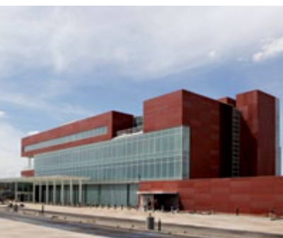
University of New Mexico Albuquerque, US | RMKM Architects Albuquerque, US | 5,850 m 2 fibreC facade | terracotta | FE, FL & MA | screwed University of New Mexico Albuquerque, US | RMKM Architekten Albuquerque, US | 5.850 m 2 fibreC Fassade | terracotta | FE, FL & MA | geschraubt
