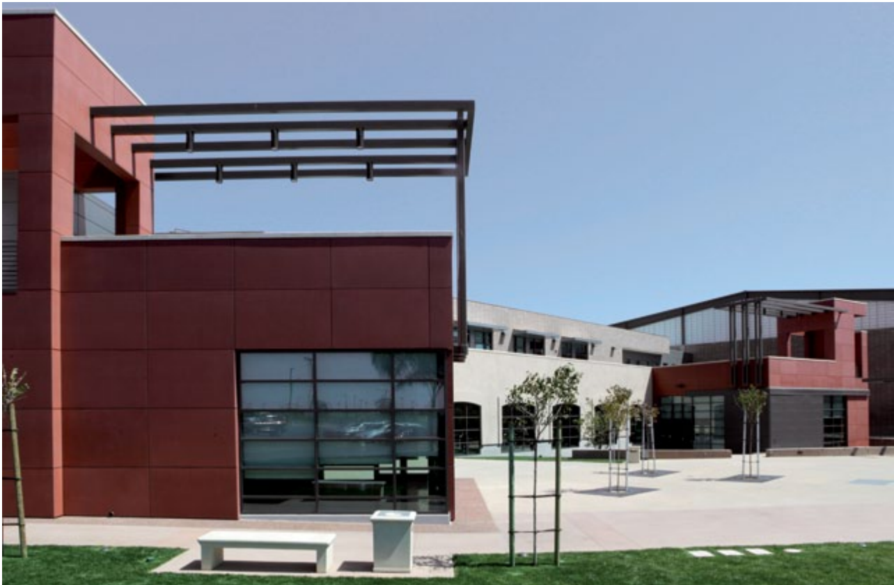
Miramar College San Diego, US | Carrier Johnson Architecture San Diego, US | 900 m 2 fibreC facade | terracotta | MA | screwed Miramar College San Diego, US | Carrier Johnson Architektur San Diego, US | 900 m 2 fibreC Fassade | terracotta | MA | geschraubt
