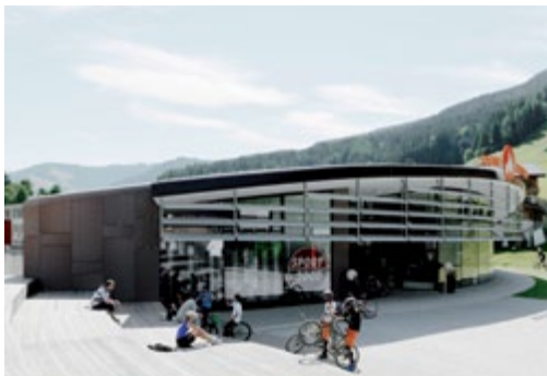
Sports Shop Mitterer, Leogang, AT | W2 Manufaktur GmbH, Leogang, AT | 600 m 2 fibreC facade | terra | FE | riveted Sportshop Mitterer, Leogang, AT | W2 Manufaktur GmbH, Leogang, AT | 600 m 2 fibreC Fassade | terra | FE | genietet
