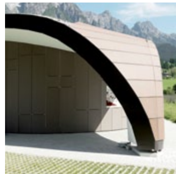
Sports Shop Mitterer, Leogang, AT | W2 Manufaktur GmbH, Leogang, AT | 600 m 2 fibreC facade | terra | FE | riveted Sportshop Mitterer, Leogang, AT | W2 Manufaktur GmbH, Leogang, AT | 600 m 2 fibreC Fassade | terra | FE | genietet
