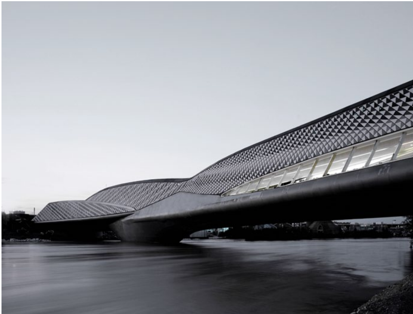
Zaragoza Bridge Pavilion for EXPO 2008 Zaragoza, ES | Zaha Hadid Architects London, UK | 11,500 m 2 fibreC facade | grey shades | FE | riveted Zaragoza Bridge Pavilion für die EXPO 2008 Saragossa, ES | Zaha Hadid Architekten London, UK | 11.500 m 2 fibreC Fassade | Grautöne | FE | genietet
