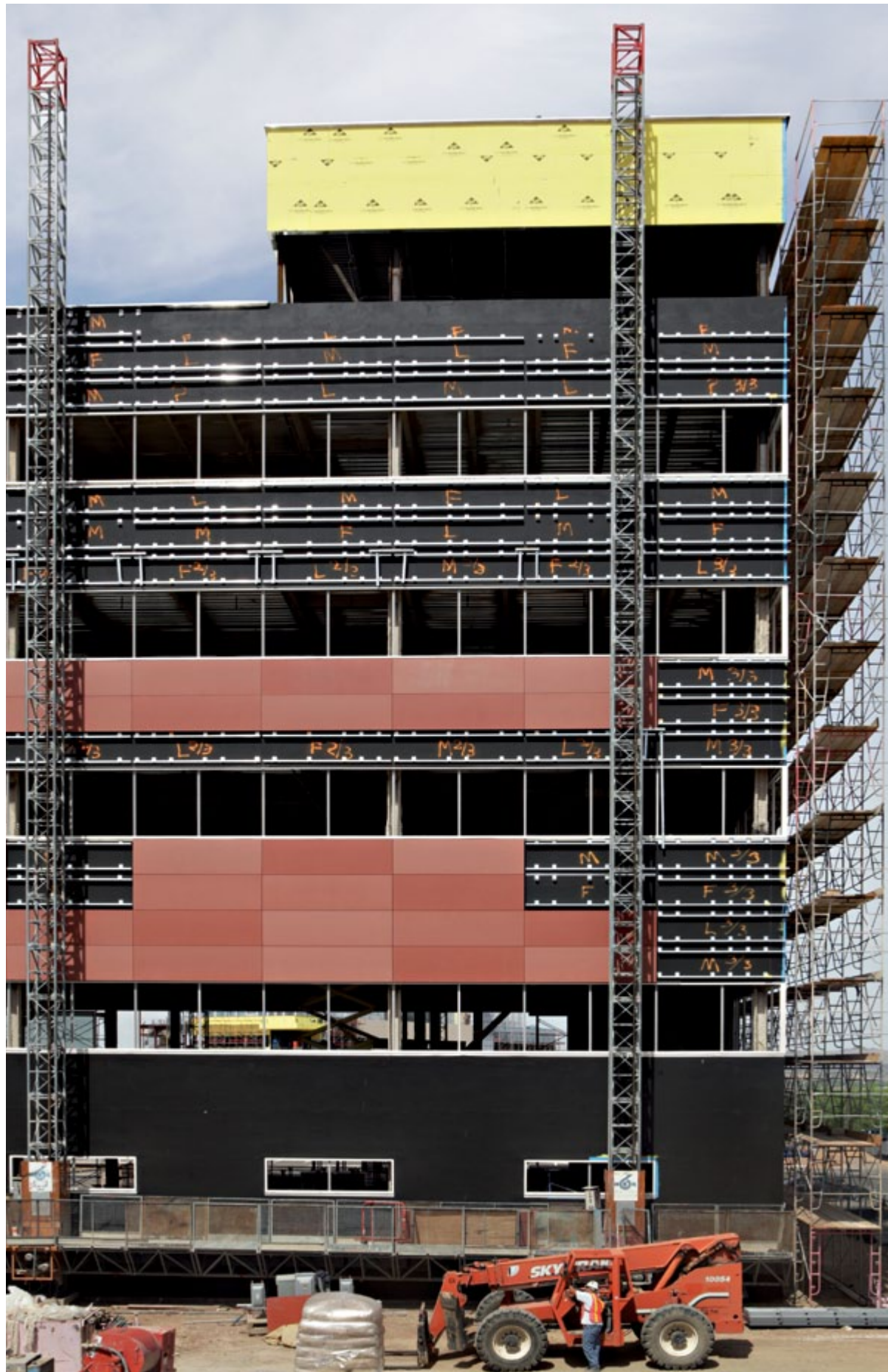
University of New Mexico Albuquerque, US | RMKM Architects Albuquerque, US | 5,850 m 2 fibreC facade | terracotta | FE, FL & MA | screwed University of New Mexico Albuquerque, US | RMKM Architekten Albuquerque, US | 5.850 m 2 fibreC Fassade | terracotta | FE, FL & MA | geschraubt
