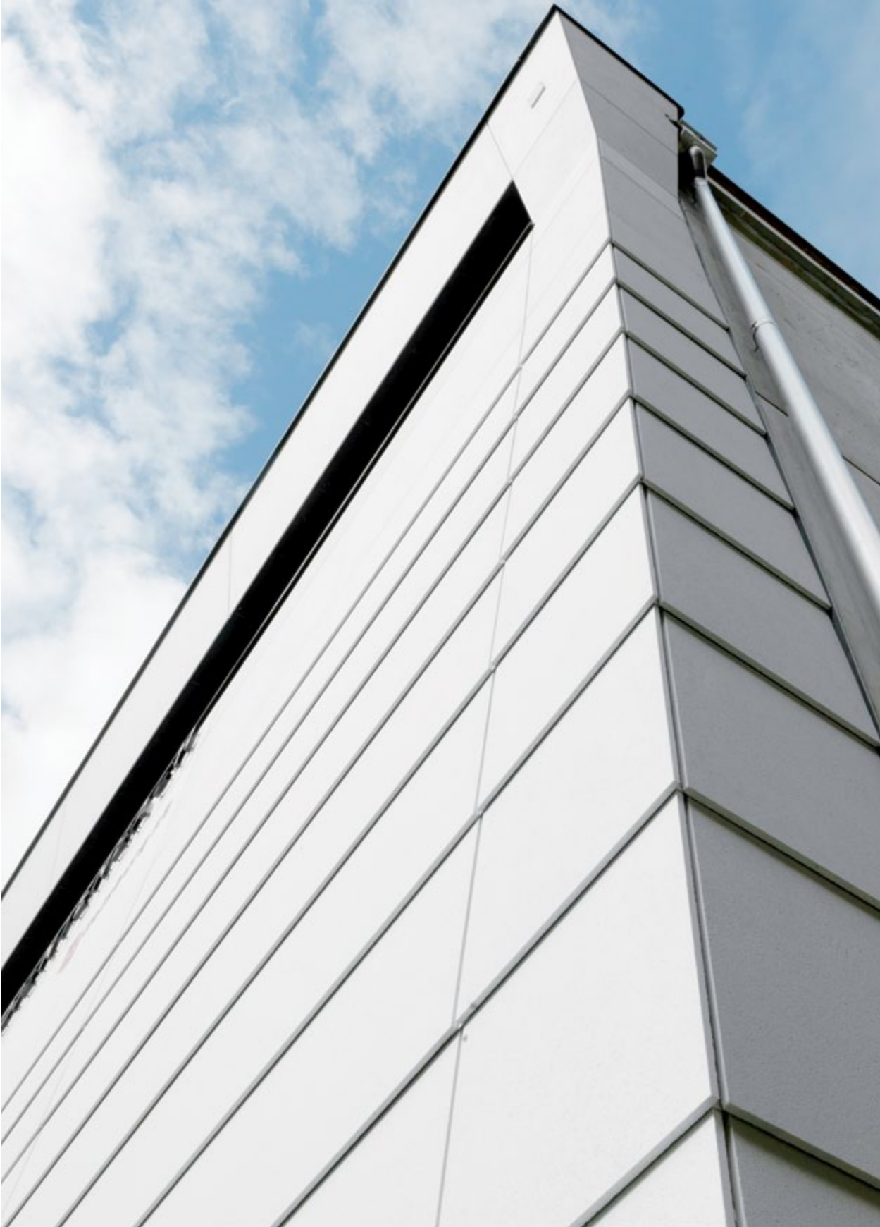
Hydropower Plant Dientenbach Lend, AT | 500 m 2 fibreC facade | bianco | FE | lap siding Wasserkraftwerk Dientenbach Lend, AT | 500 m 2 fibreC Fassade | bianco | FE | Stülpchalung
