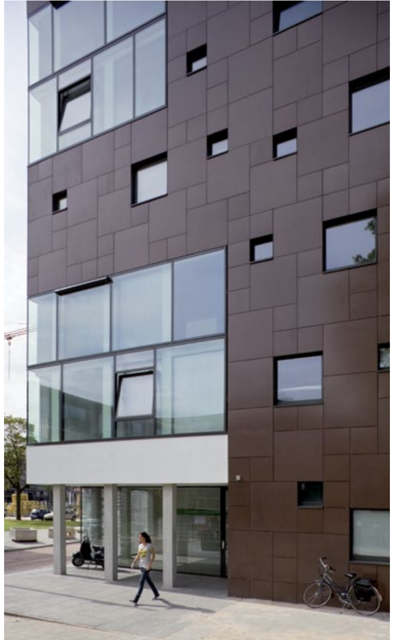
Dormitory Blok 1 Presikhaaf Arnhem, NL | Group A Rotterdam, NL | 1,900 m 2 fibreC facade | terra | FE & FL & MA | screwed Studentenwohnhheim Blok 1 Presikhaaf Arnhem, NL | Group A Rotterdam, NL | 1.900 m 2 fibreC Fassade | terra | FE & FL & MA | geschraubt
