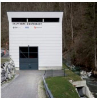
Hydropower Plant Dientenbach Lend, AT | 500 m 2 fibreC facade | bianco | FE | lap siding Wasserkraftwerk Dientenbach Lend, AT | 500 m 2 fibreC Fassade | bianco | FE | Stülpchalung
