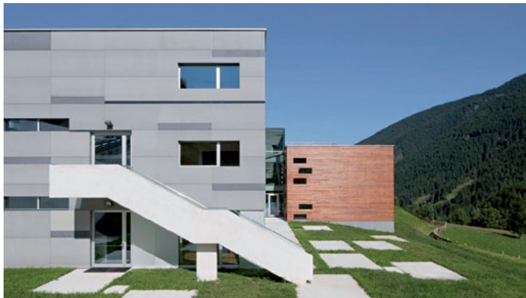
Primary School St. Walburg, IT | S.O.F.A. Architects Vienna, AT | 1,200 m 2 fibreC facade | silvergrey & anthracite | FE | riveted Grundschule St. Walburg, IT | S.O.F.A. Architekten Wien, AT | 1.200 m 2 fibreC Fassade | silbergrau & anthrazit | FE | genietet
