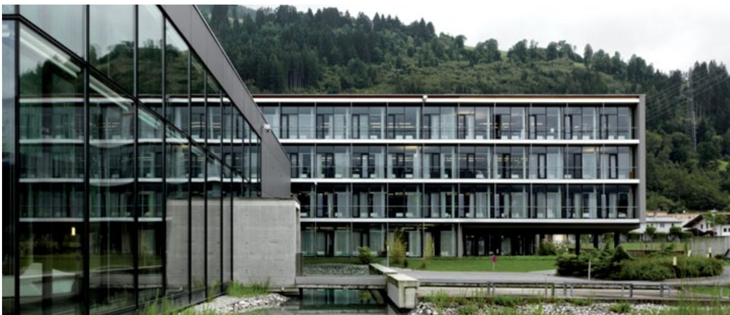
Hydropower Plant Neubruck Scheibbs, AT | Juland Barcelona Vienna, AT | 550 m 2 fibreC facade | anthracite | FL & MA | riveted Kraftwerk Neubruck Scheibbs, AT | Juland Barcelona Vienna, AT | 550m 2 fibreC Fassade | anthrazit | FL & MA | genietet
