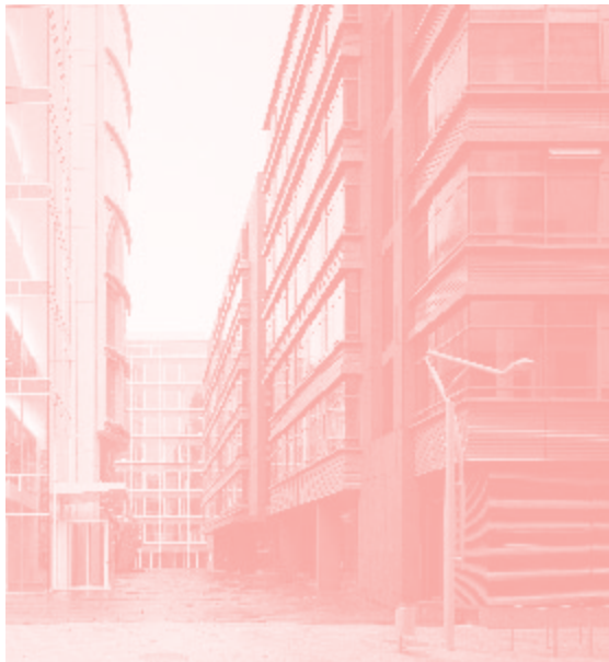
Bavaria Office Hamburg, DE | Axthelm Architects Potsdam, DE | 1,900 m 2 fibreC facade | ivory | MA | undercut anchors Bavaria Office Hamburg, DE | Axthelm Architekten Potsdam, DE | 1.900 m 2 fibreC Fassade | elfenbein | MA | Hinterschnittanker
